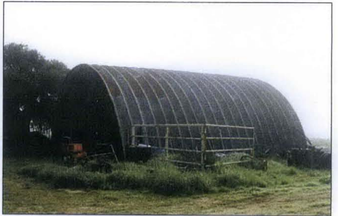
PHOTO 14: Metal storage building.
