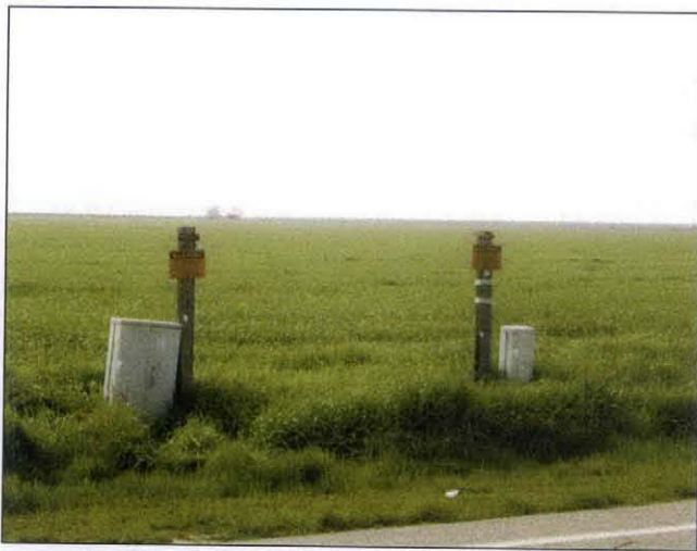
PHOTO 39: Photo showing markers for the buried telephone cables along the northern border of the Subject Property along Avenue 18.
