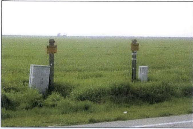
PHOTO 16: Photo showing markers for the buried telephone cables along the northern border of the Subject Property along Avenue 18.
