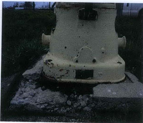
Photo 3: A second onsite well prior to well cap being secured.
