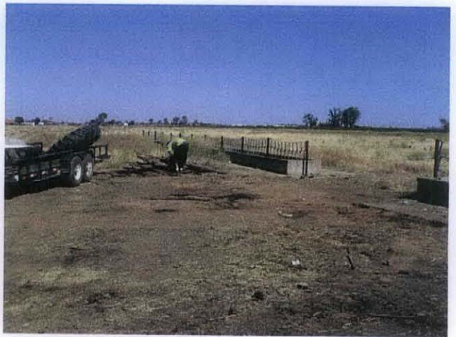
Photo 4: Photo showing equipment removal. Minimal soil staining was evident.
