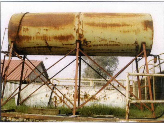
PHOTO 35: Photo showing an approximate 500-gallon gasoline above ground storage tank. The tank belongs to the current tenant occupying the Subject Property.
