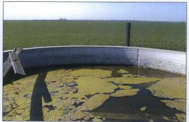
PHOTO 10: Close-up of the cistern in photo 9, showing standing water.
