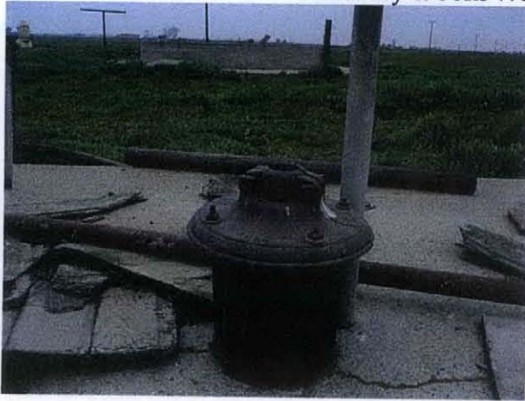
Photo 1: Photo showing onsite well prior to well cap being secured
