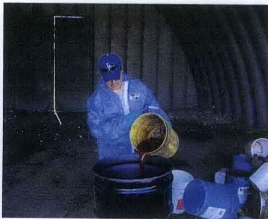
Photo 7: Proper containment of waste oil prior to removal.
