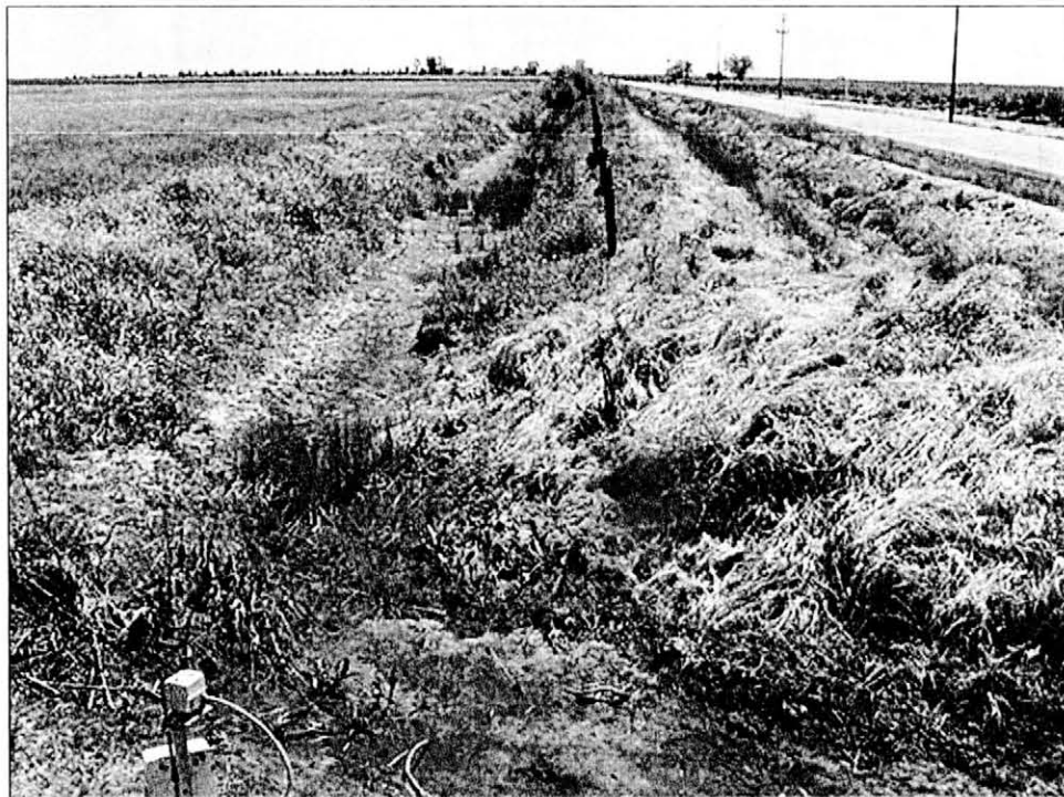
Photo 4. South view of the Schmidt Creek channel (left) and the adjacent Airport Ditch (right), along Road 23. The Airport Ditch is siphoned under the creek through a buried concrete in the right hand side of the photo. Thus, the two features are not contiguous. Note the freshwater emergent vegetation growing in an area of sand deposition just upstream.
