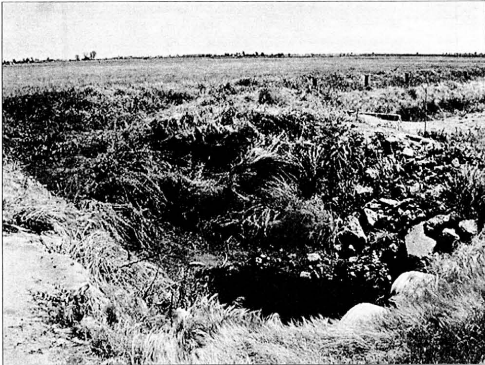
Photo 5. Southeast view of the Schmidt Creek channel as it enters the culverts under Road 23. The headwall of the concrete vault siphon of the Airport Ditch is located in the upper-middle right hand corner of the photo.
