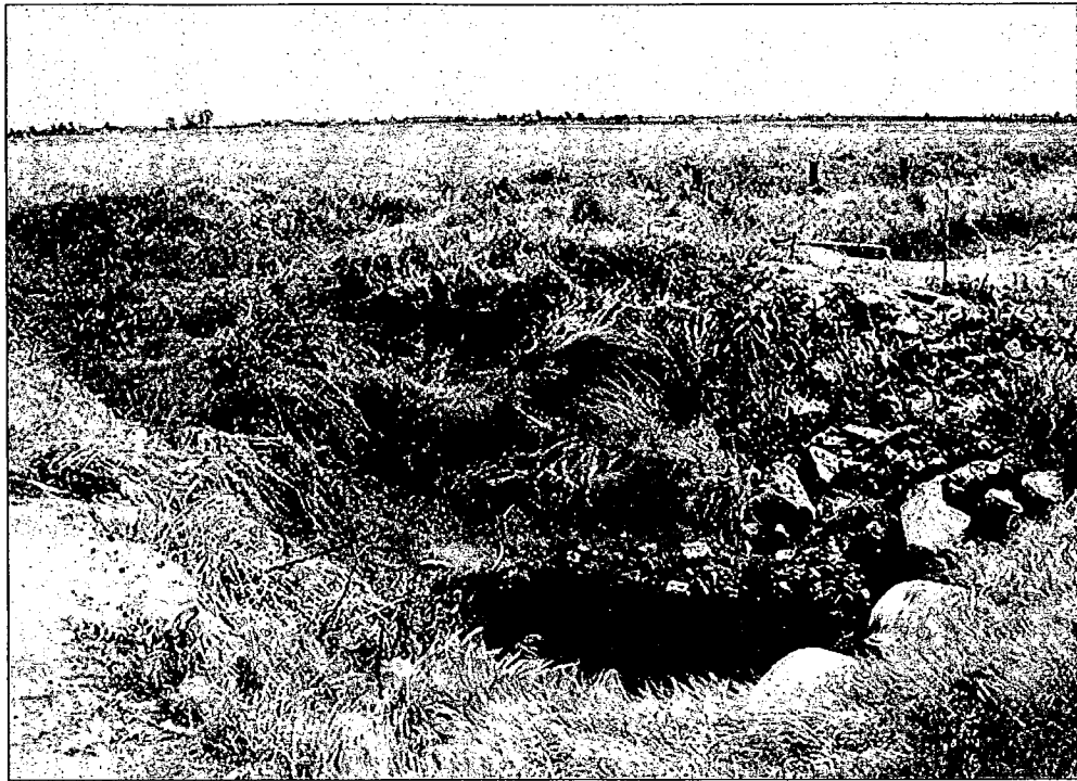
Photo 5. Southeast view of the Schmidt Creek channel as it enters the culverts under Road 23. The headwall of the concrete vault siphon of the Airport Ditch is located in the upper-middle right hand corner of the photo.
